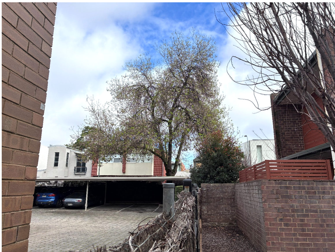
Figure 3.7 – Adjacent site to south viewed from the east
